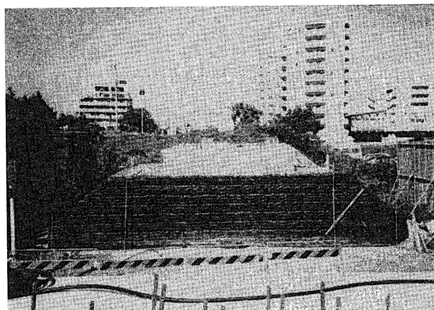
Photo 6. Abutment before casting-in-place facing
